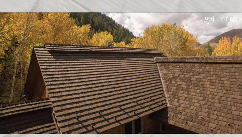
safety standards. The prospect that there could be natural and realistic looking synthetic shakes that meet Class A (combustible material) fire standards seemed too good to be true. That is, until local roofing expert Miley found a replacement product that made it possible to have the look of a traditional hand-split cedar shake roof with up-to-date fire protection. "We have been installing them as new roofs and roof
