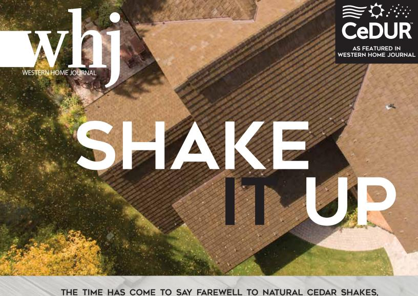
THE ROOFING MATERIAL SO COMMON TO THE WOOD RIVER VALLEY AND THE ENTIRE UNITED STATES. IT IS SIMPLY TOO FLAMMABLE FOR THE HIGH MOUNTAIN DESERT. IN RESPONSE, SCOTT MILEY ROOFING HAS TEAMED UP WITH CEDUR TO INSTALL POLYURETHANE SYNTHETIC SHAKE ROOFS THAT MEET FIRE SAFETY STANDARDS WHILE MAINTAINING A TRADITIONAL LOOK THAT IS DIFFICULT TO DISCERN FROM WOOD. Scott Miley Roofing (SMR) has been building and replacing roofs in
